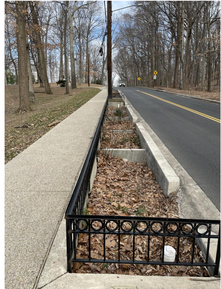
Oregon Ave drainage structure along Oregon Avenue NW, Source: DDOT
